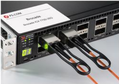
Brocade ICX 7750-26Q
