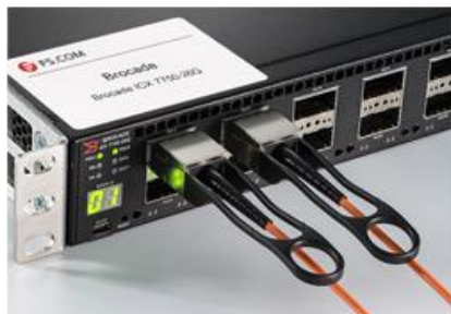
Brocade ICX 7750-26Q
